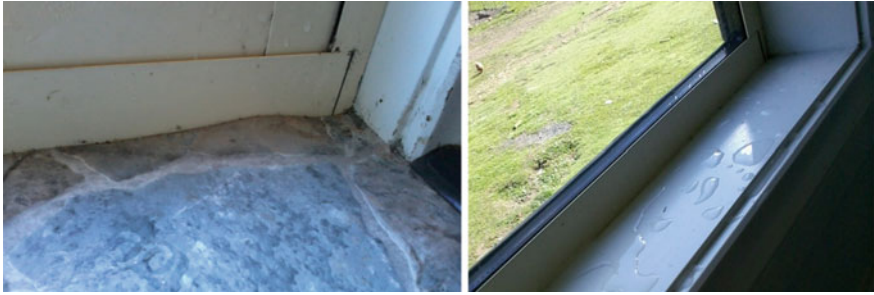
Fig. 19 Condensation forming on the kitchen flooring due to poorly installed insulation and a vapour impermeable vinyl finish. Around the window reveals the thermal bridging of the structure results in condensation
