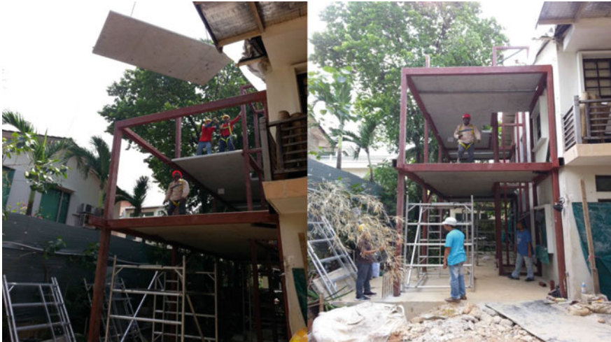
Fig. 6 Lifting and placing of pre-cast slabs onto modules
