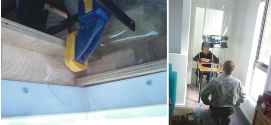
Fig. 11 Blower door apparatus modified for testing roof cavity
