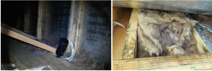
Fig. 21 Under the bed, the wall and carpet have limited exposure to the heating and experience thermal bridging to the external walls
