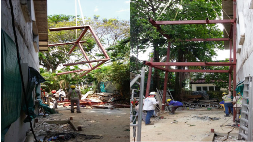
Fig. 5 Lifting and installing onto pre-fixed sleeves of first module on site
