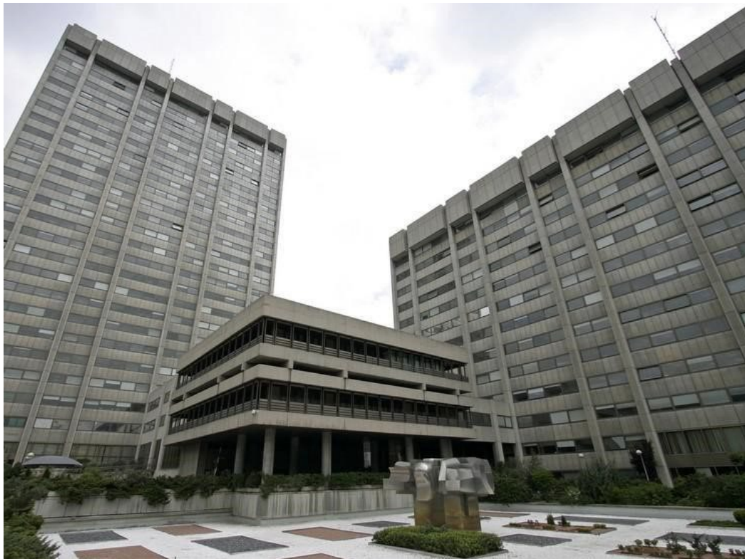
Figure 15: Public building, Spain (Picture provided by Carlos Barcena, Dragados)
