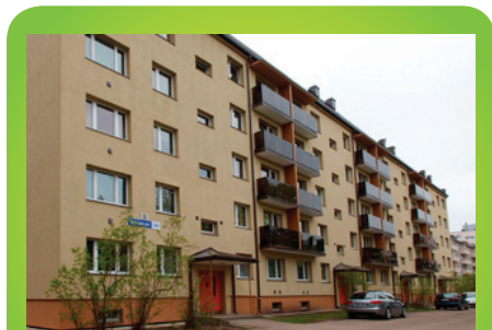
Refurbishment work using KredEx fund
