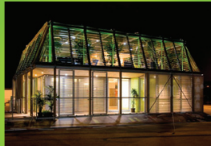
Top floor of the nanotower with communal space beneath the solar canopy roof
