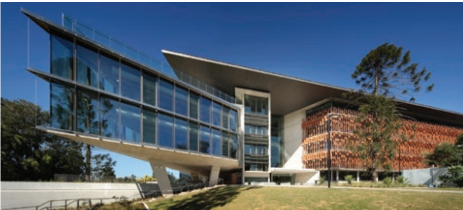
University of Queensland Advanced Engineering Building, Brisbane QLD, designed by CRCLCL participant HASSELL.
