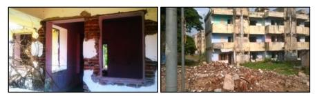
Window and Door Frames Being Removed Before Demolition (Left) and Demolition Site of TNHB Housing Units (Right)
