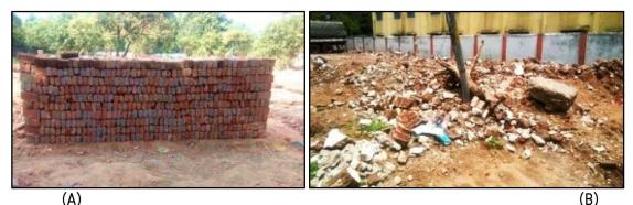
Figure 15: (A) Segregation of Whole Bricks on Site; (B) Illegal Dumping on the Road
