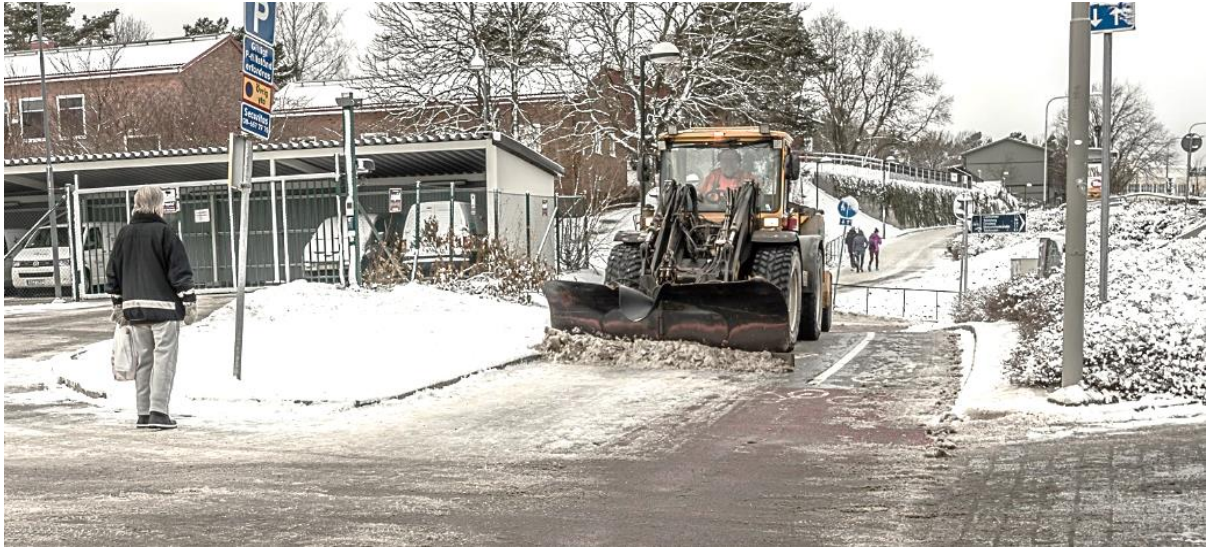
Figure 7. Snow clearing of a walking and cycling path. Photo: Göran Blomqvist, VTI.
