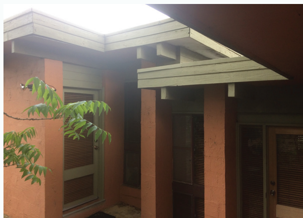
Figure 6. Exterior of house before renovation (Image: Cooee Architecture)
