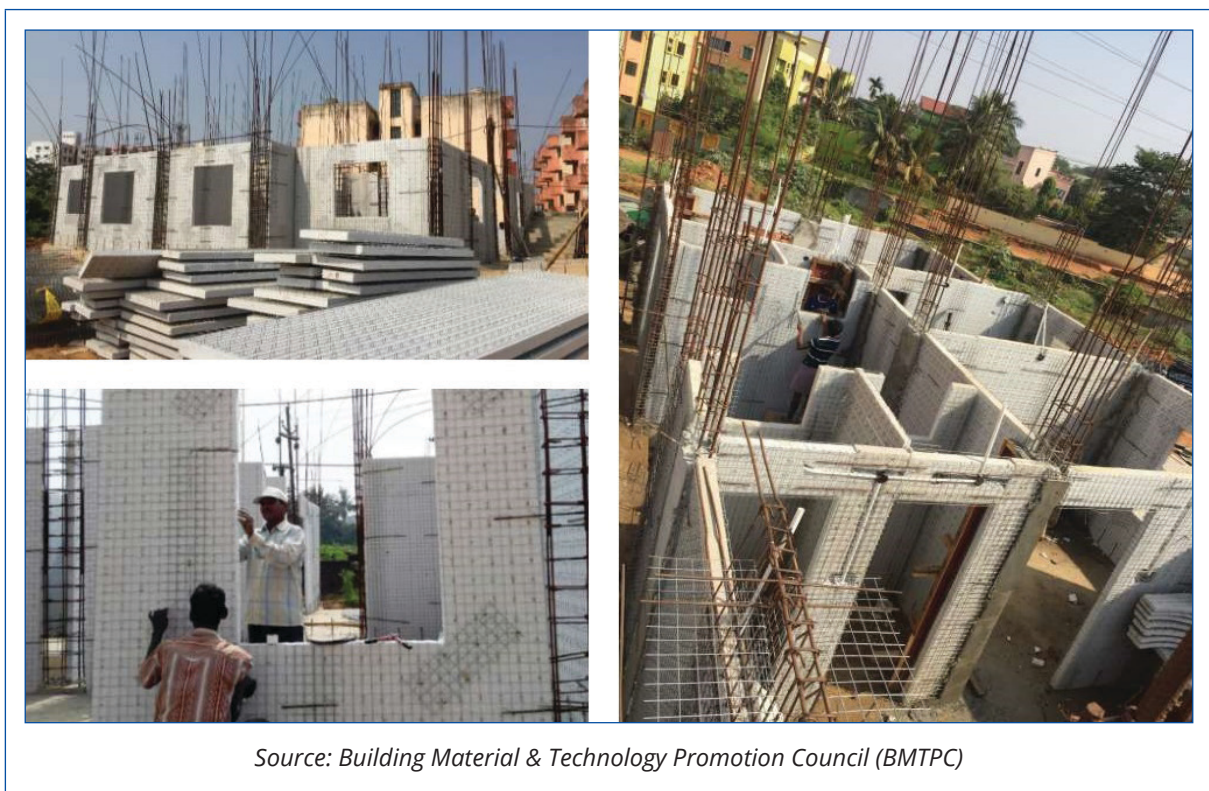
Figure 10: Prefabricated construction – EWS housing in Chandrashekharpur
