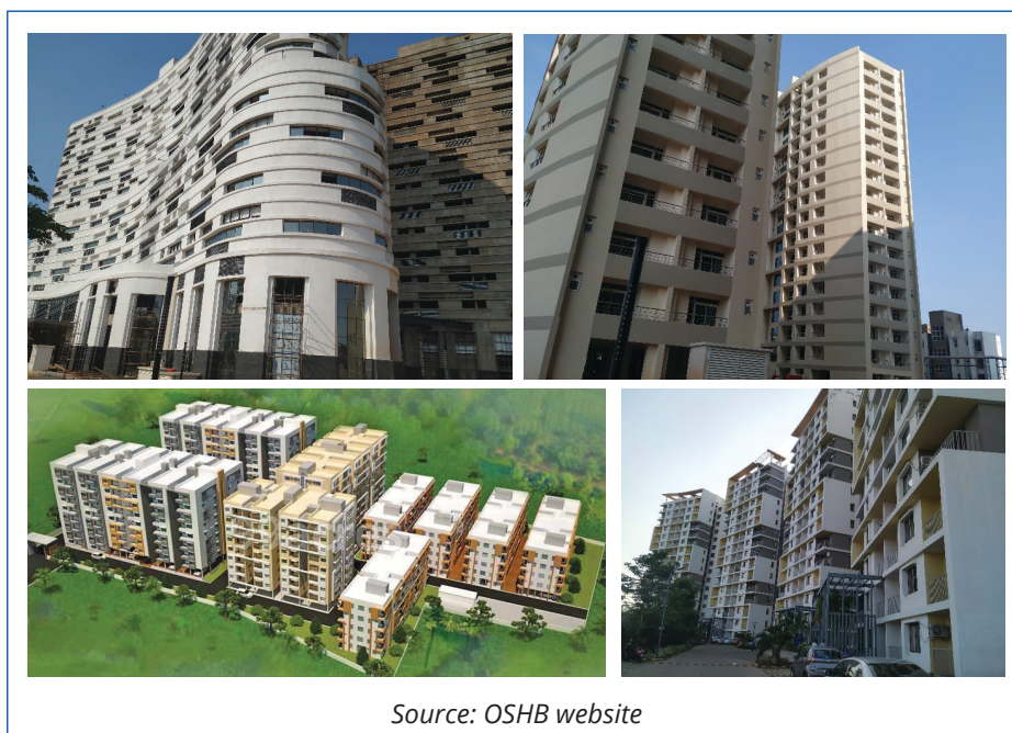
Figure 7: High rise residential construction in Bhubaneswar
