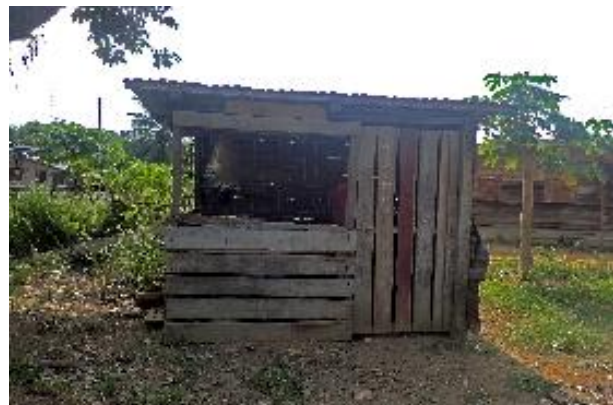
Photo 5: One of the storage facilities witnessed during the assessment of effectiveness of intervention model
