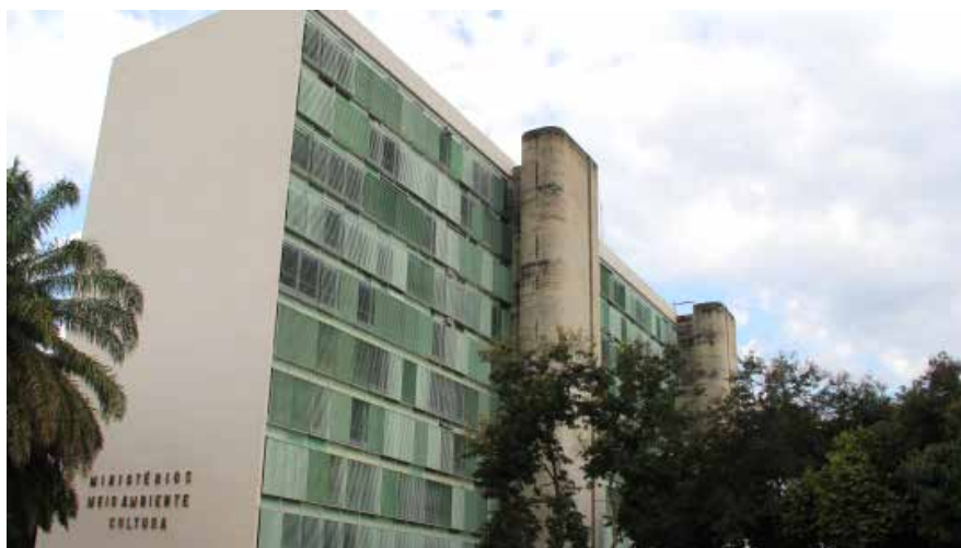
The B block of the Esplanade of Ministries, which houses the Ministries of Environment and Culture, will serve as a model of energy efficiency for other public buildings
