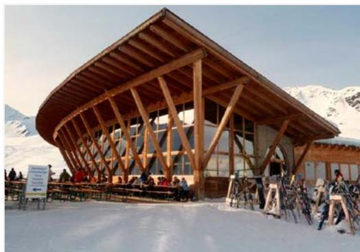
The Skirestaurant Masner located at Serfaus in Tirol invested in energy efficiency through the installation of 120m<sup>2</sup> solar panels support the heating of water and room air. Together with a highly insulated envelope of the building and a ventilation system with heat recovery, the annual heating requirement is reduced to a quarter compared to a conventional building.
