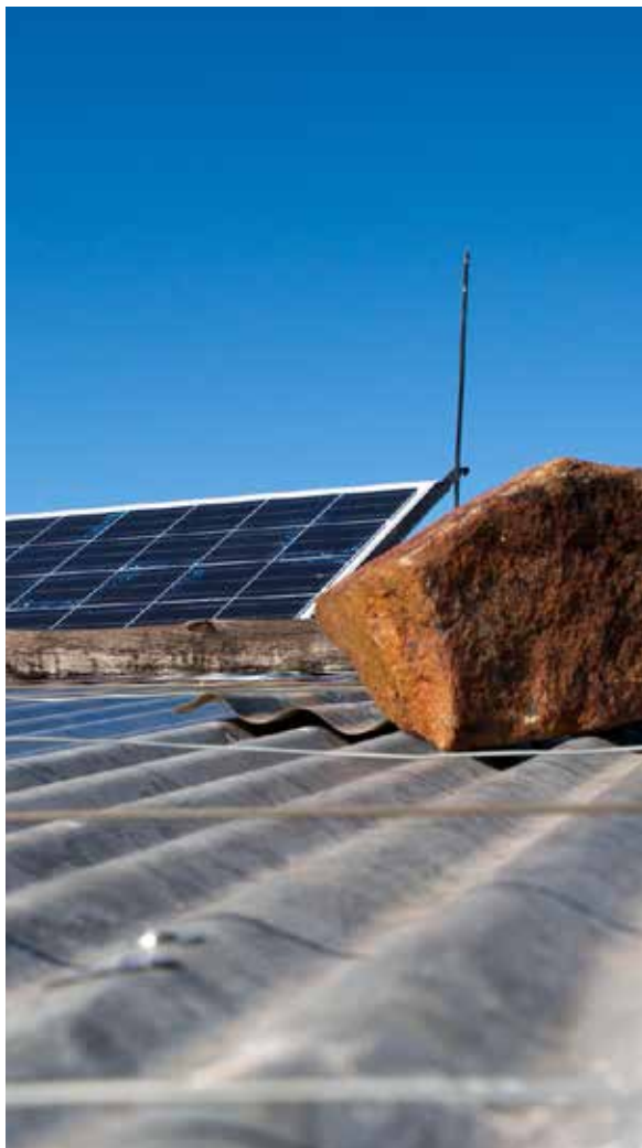
© Specialized Solar Systems
