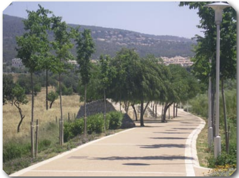
Paseo de Calvià, pathway linking urban and rural settlements, lit by solar energy
