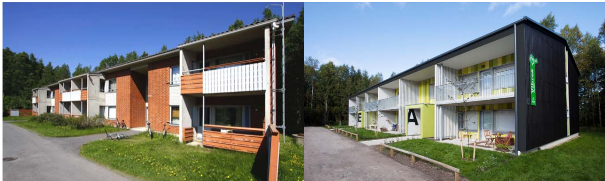
Figure 3: Oulu demonstration before retrofit in 2011 and at completion in 2013 (photos M3 Architects)
