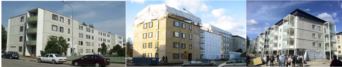
Figure 29: Riihimäki Innova project before TES retrofit, during facade assembly, and completed (S. le Roux 2011-2012)
