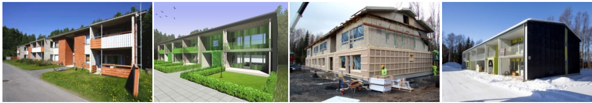
Figure 6: Building in 2011, design stage 2012, TES assembly phase in 2012, and completed in 2013 (photos M3 Architects)
